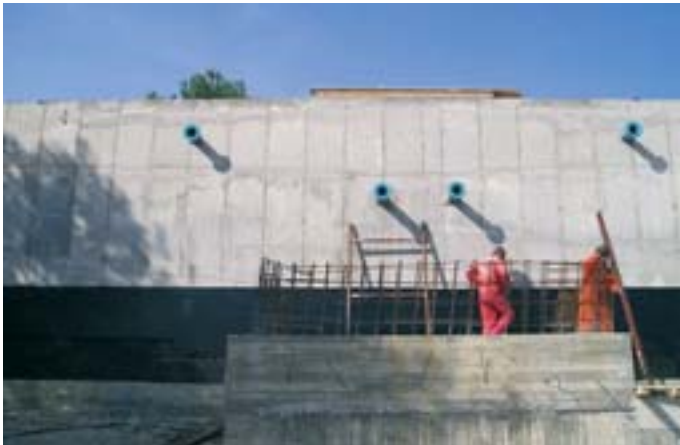
Work in progress: water storage construction site, Gjirokaster
