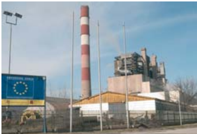
Nikola Tesla A power station, Obrenovac
