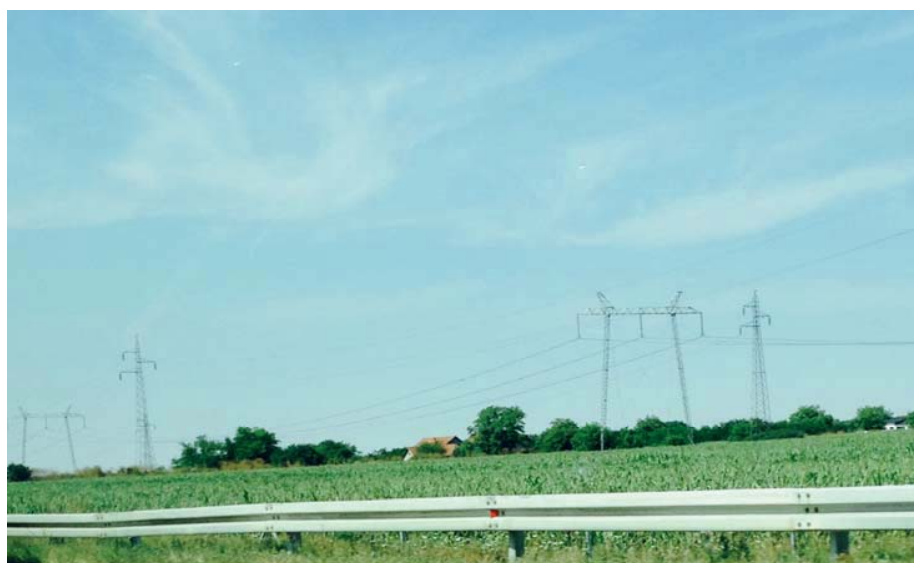
View of existing 110 and 400 kV transmission lines.
