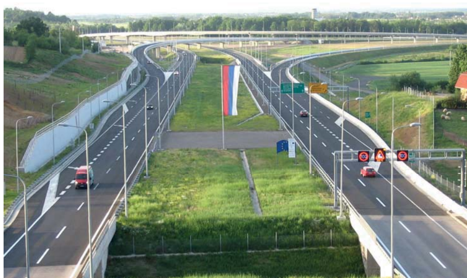
Upgraded interchange in Mahovljanska, Bosnia and Herzegovina.
