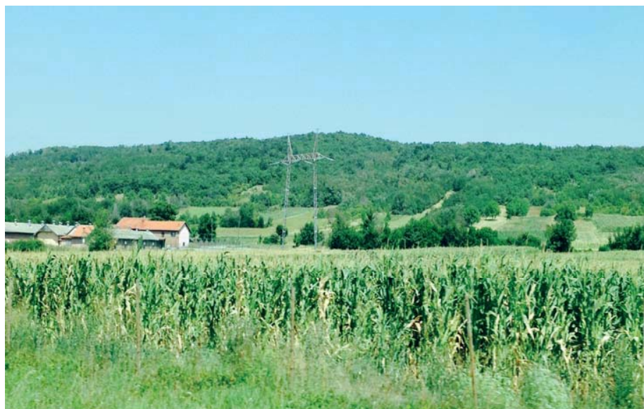
View of existing 400 kV transmission lines along the Trans-Balkan Corridor.
