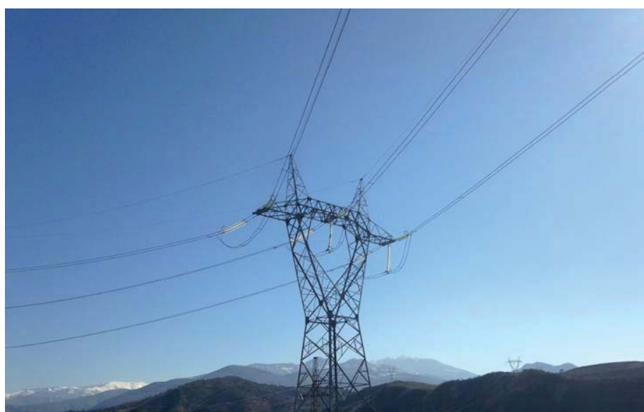
Existing 400 kV transmission lines in Elbasan, Albania.
