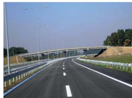
View of Banja Luka – Gradiška motorway, Bosnia and Herzegovina.
