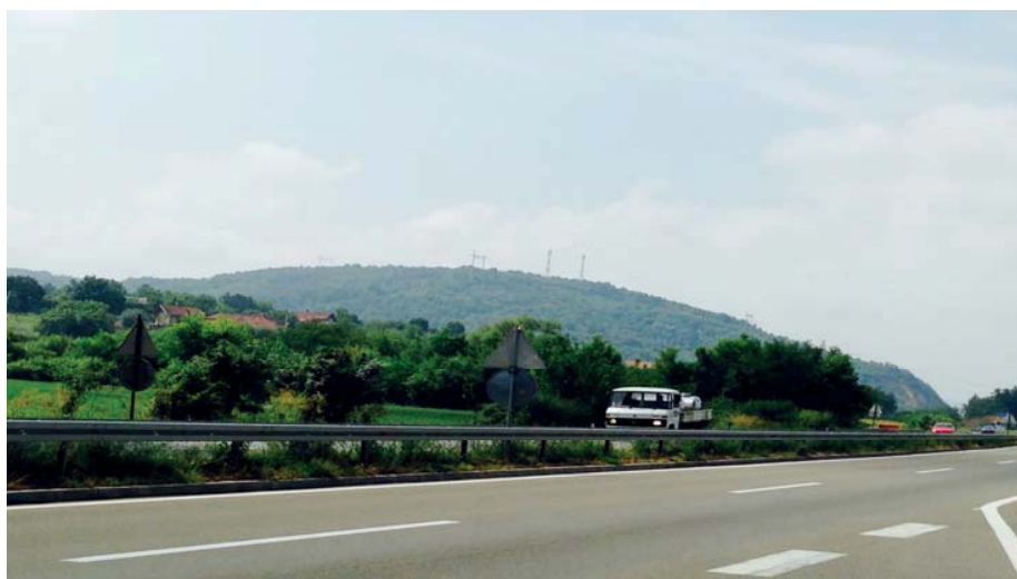
View of existing 400 kV transmission lines in Kragujevac.
