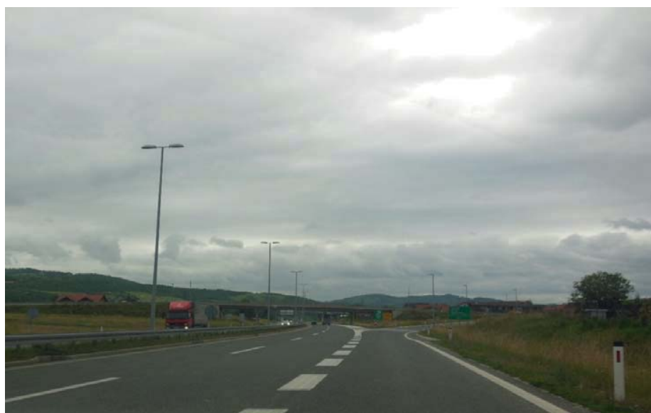
Upgraded interchange on Corridor Vc, Bosnia and Herzegovina.
