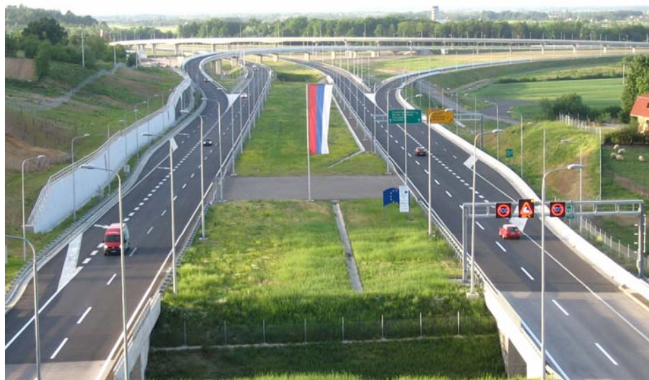
Upgraded interchange in Mahovljanska, Bosnia and Herzegovina.
