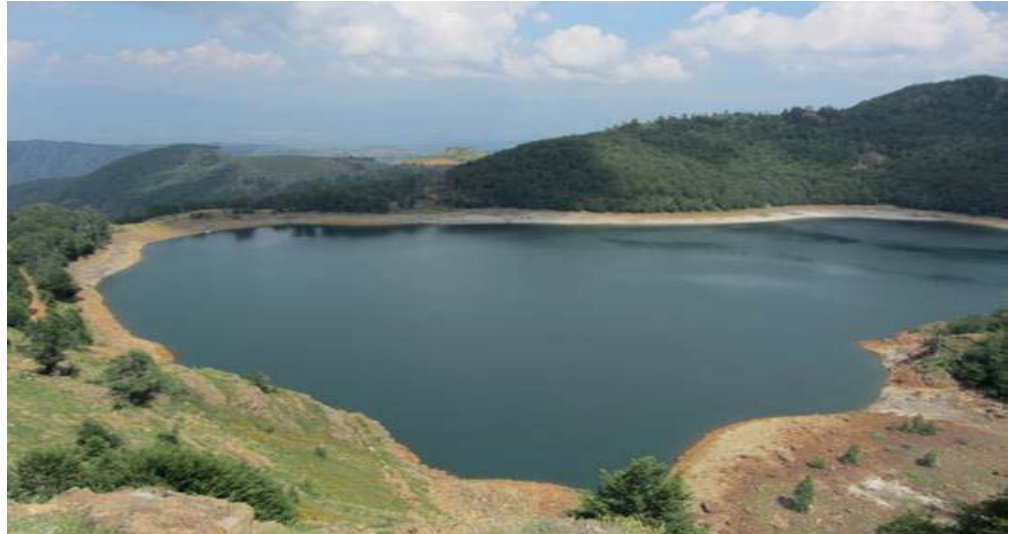
Ternoves Hydropower Plant, Albania
