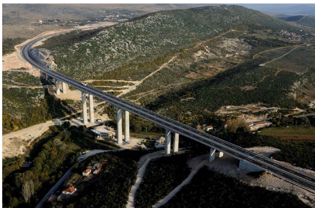
Existing motorway on Corridor Vc in Bosnia and Herzegovina.
