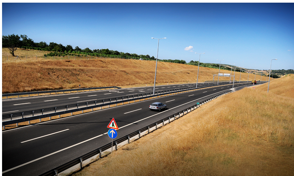
Existing motorway on Route 7 in Kosovo.
