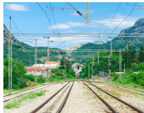
Electrified rail along Bar – Vrbnica.
