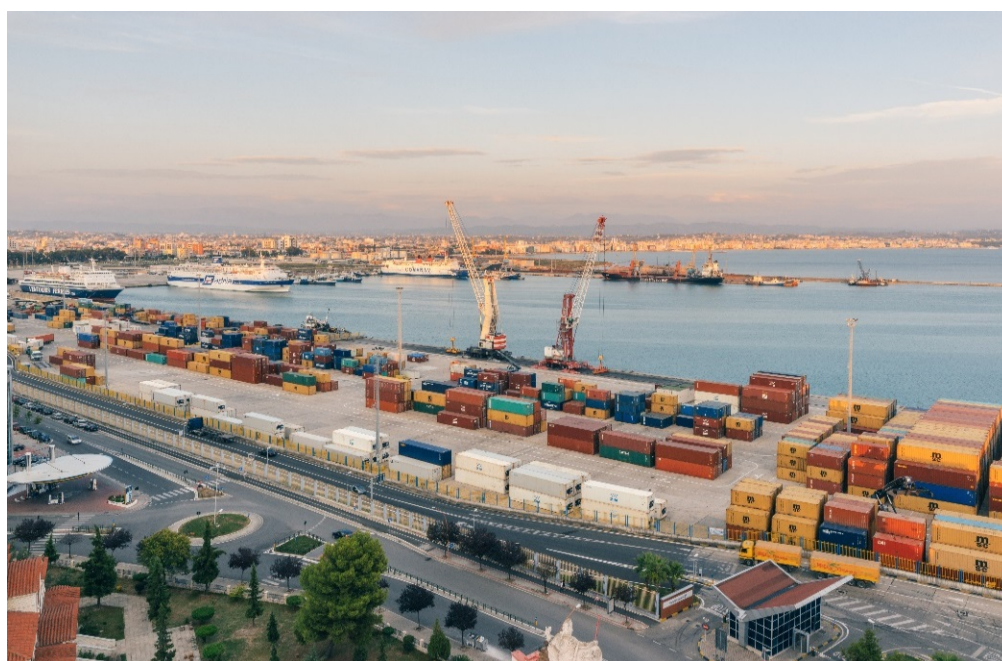
View of Durrës Port, container/logistics area.
