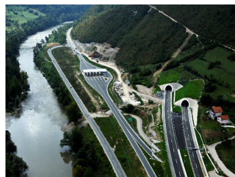
Corridor Vc in Bosnia and Herzegovina.
