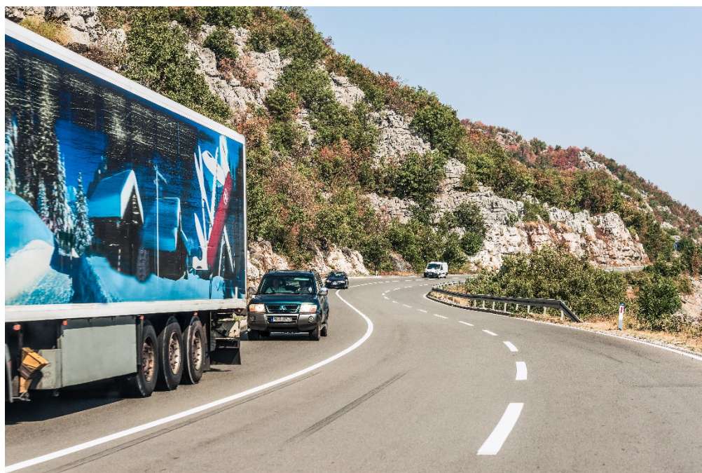
Existing road to Budva, on the Adriatic-Ionian Expressway (R1).
