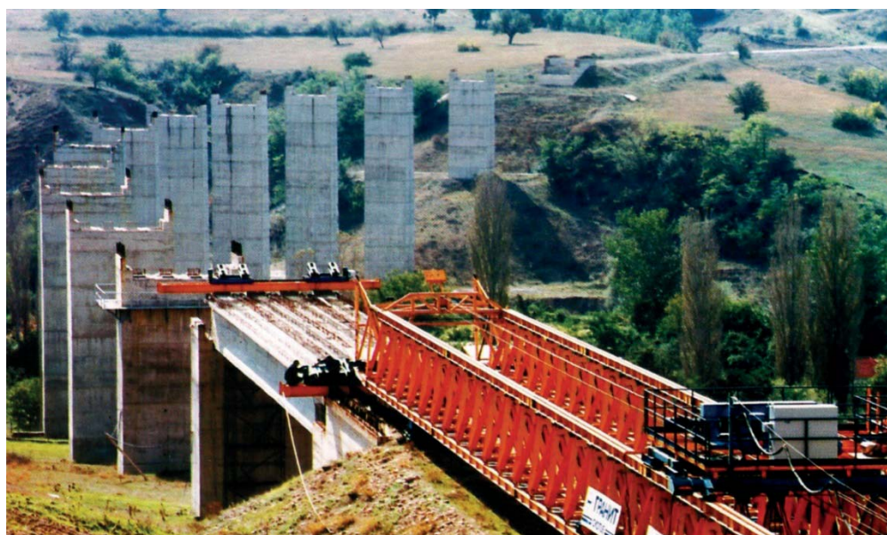
View of railway track construction works on Kumanovo – border with Bulgaria railway section, the former Yugoslav Republic of Macedonia.
