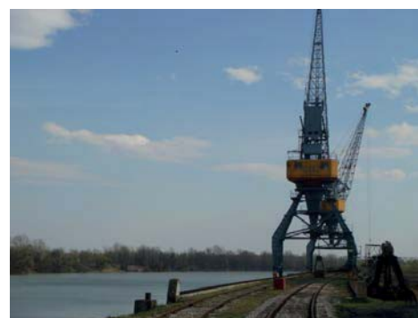
Existing harbor crane and associated railway track in the Port of Brčko.
