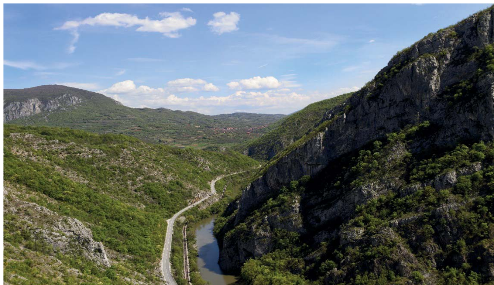
View of non-electrified railway track (as well as two-lane road) in Sićevo Gorge, on Corridor Xc, Serbia.
