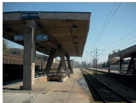
Train station in Niš on Corridor X, Serbia.
