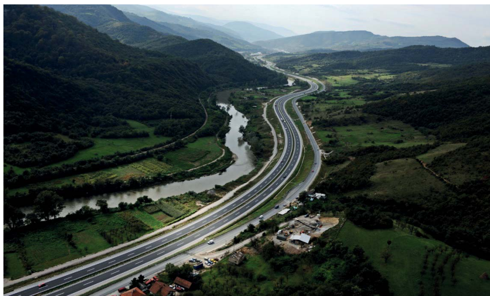
Newly built motorway on the Tarčin – Sarajevo – Zenica section on the Mediterranean Corridor in Bosnia and Herzegovina.
