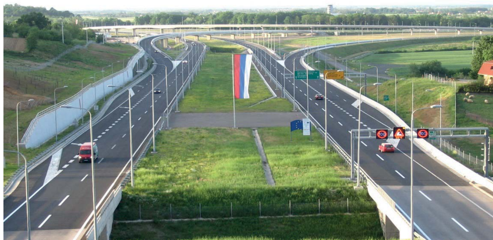
Newly built Mahovljani Interchange on the Banja Luka – Dobož motorway in Bosnia and Herzegovina.
