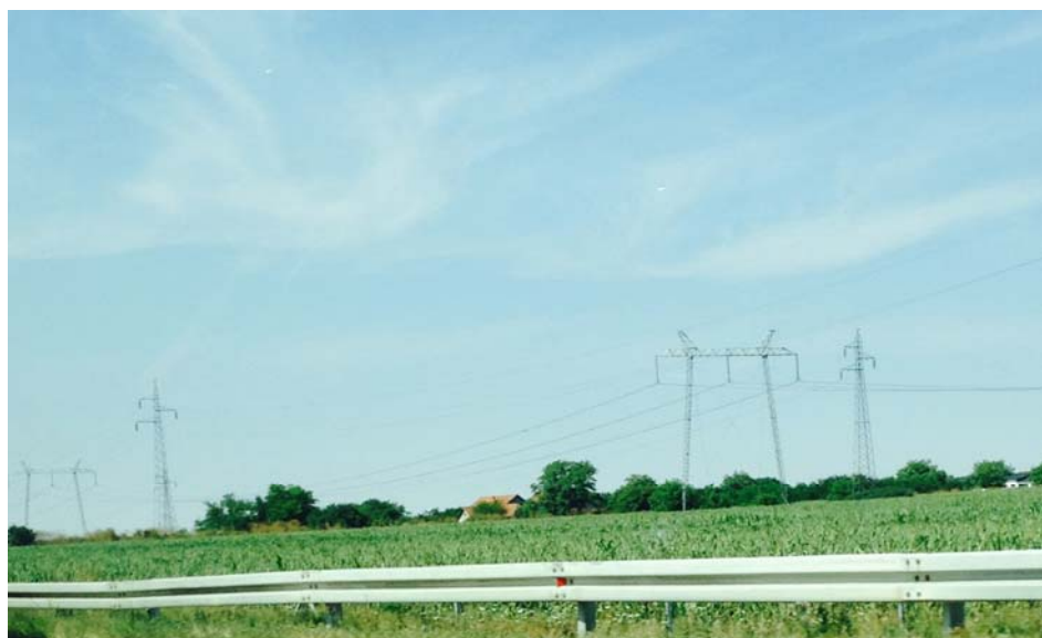
View of existing 110 and 400 kV transmission lines.
